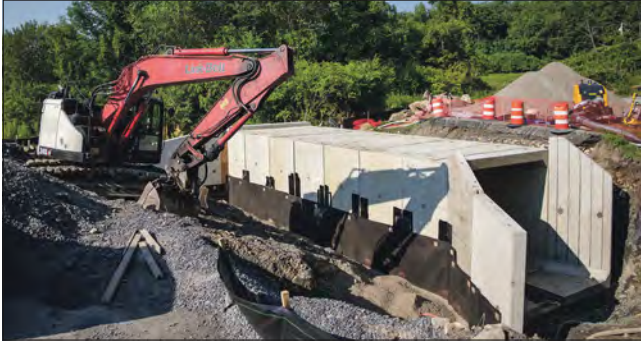
PHOTO BY NATHAN MILLER The new concrete culvert will carry the Shekomoko Creek under Route 199.
