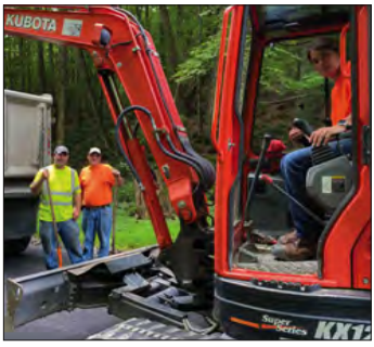
AMENIA Tower Hill Road paving A3
