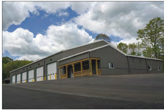
New facility on Route 22 is nearly finished. Plans call for moving into the new building in the first week of June.
