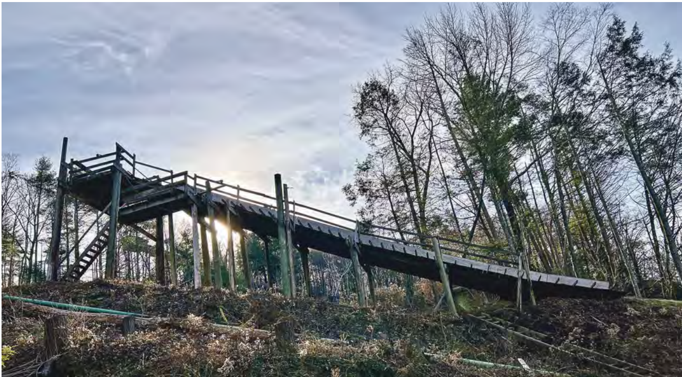
Profile of the existing 30 Meter tower erected nearly 75 years ago!
