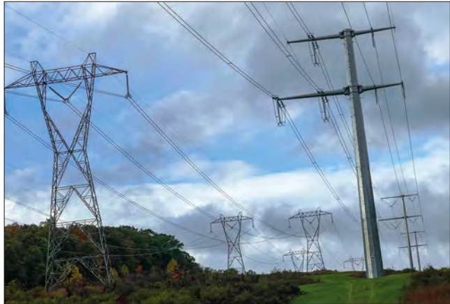
Power transmission lines cross Route 199 east of Rhinebeck.
