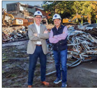
MILLBROOK Demolition Begins On Bennett Park Project A3
